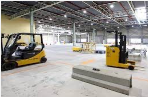
Factory Machinery Localization Algo
